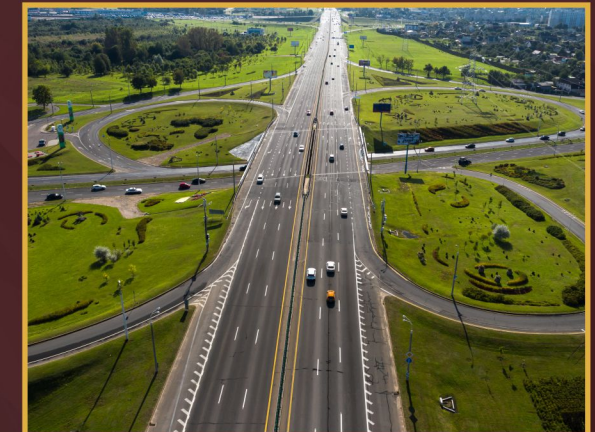
KGP/KMP Expressway Eastern/Western Peripheral Expressway
