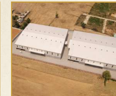
2026 SVG Warehouse-2 Noida International Airport Road, Greater Noida
